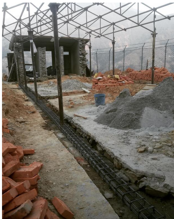
Adding foundations for Shree Dhanjala Basic School
